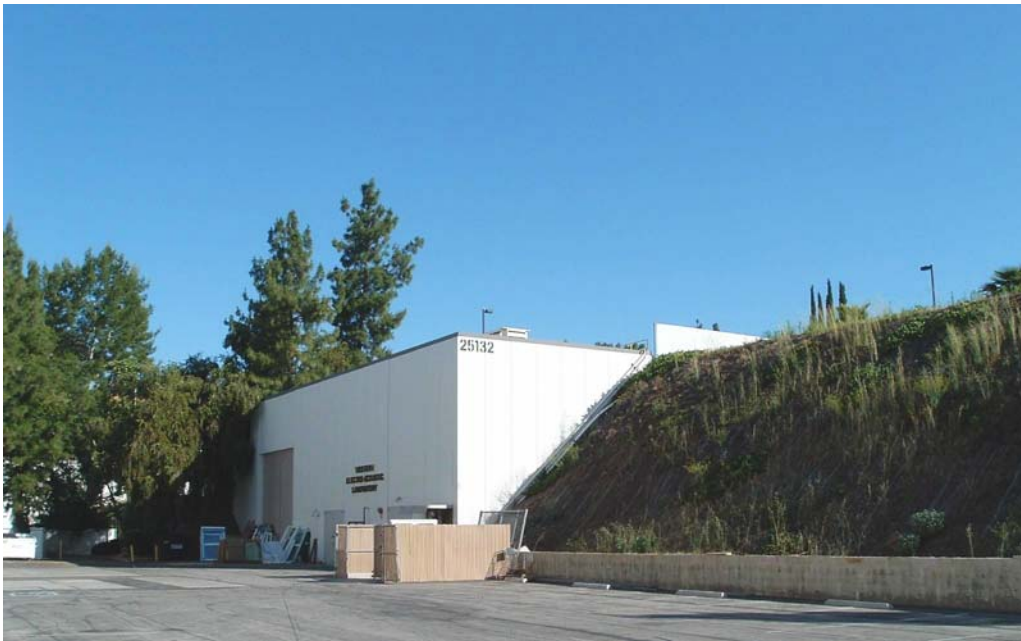
Photo 2 – Exterior of the building in which the anechoic chamber is located
